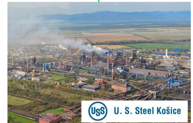
6. Steel producer U.S. Steel Košice, s.r.o & EASTGATE H 2 Valley
